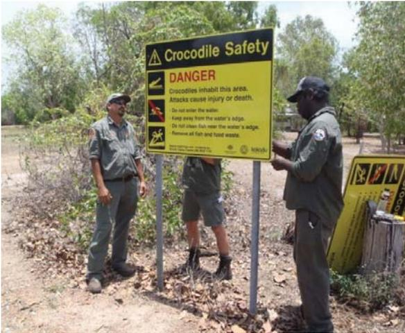
The Kakadu Signage Project is progressing with the first new signs in the ground. Rangers were trained on 5 November in sign installation specifications. Rangers of course know how to dig a hole and mix concrete! The training goes a step further, with instructions based on Australian Standards, specifying post heights, hole depths and sign placement to ensure consistency across the park.
