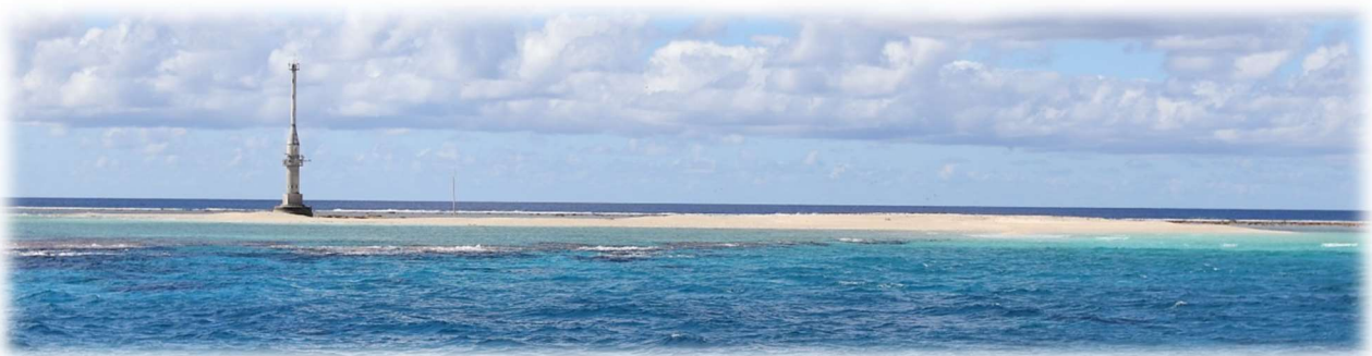
Photo 97 The 33m tower at Lighthouse Cay
